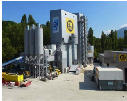
Figure 10: Illustration of the central installed by Marti on the Champel working site
